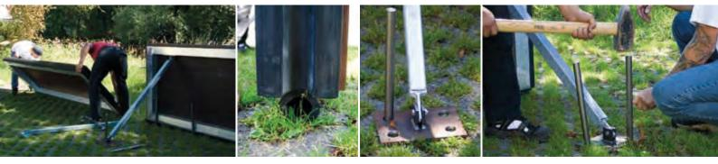
On a naturally grown surface the wall support is secured with steel needles.
